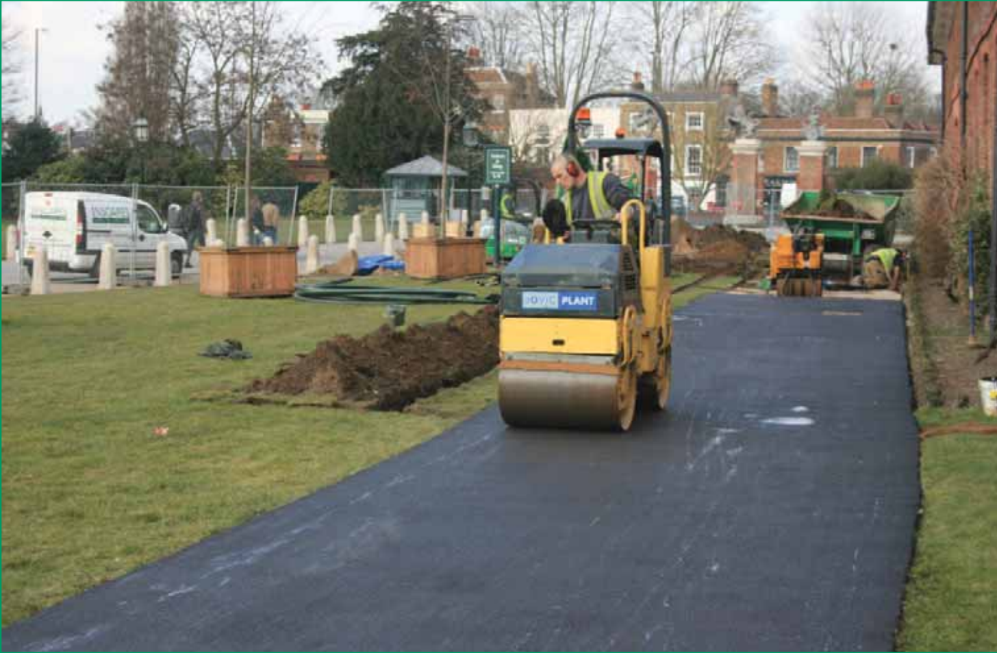
Tarmac was layed with a resin-bonded surface along these pedestrian routes.
